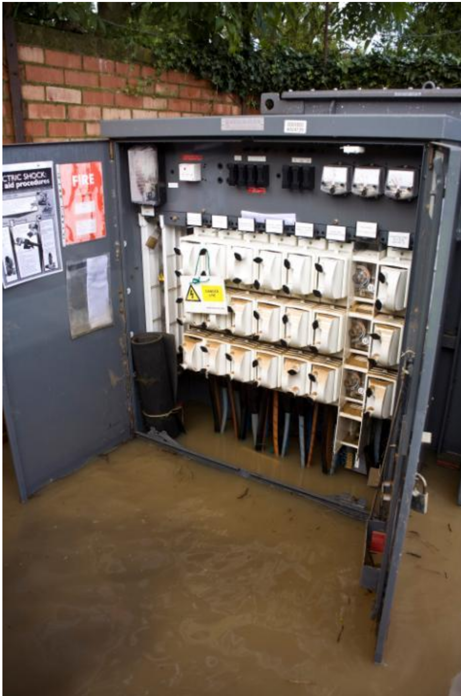
Photograph 5 – The low-voltage fusegear at Brown's Bridge Distribution Substation
